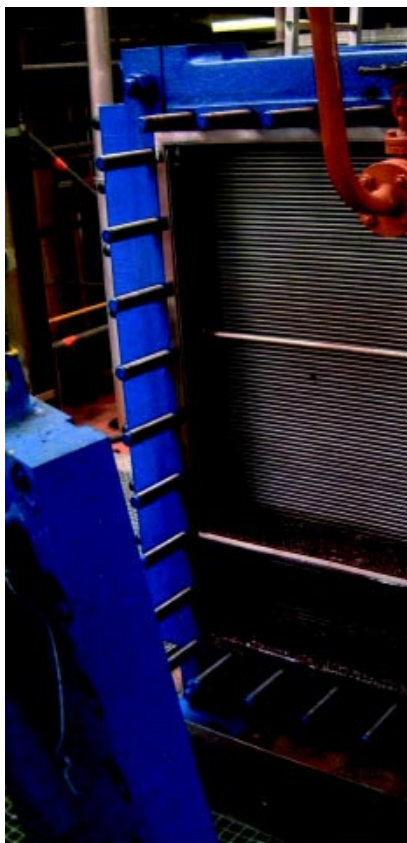
Fig. 8 Photo showing before and after high-pressure water-jet cleaning of the cooling water circuit of a CPHE operating as condenser in the solvent recovery part of a paraffin removal plant in Europe.
