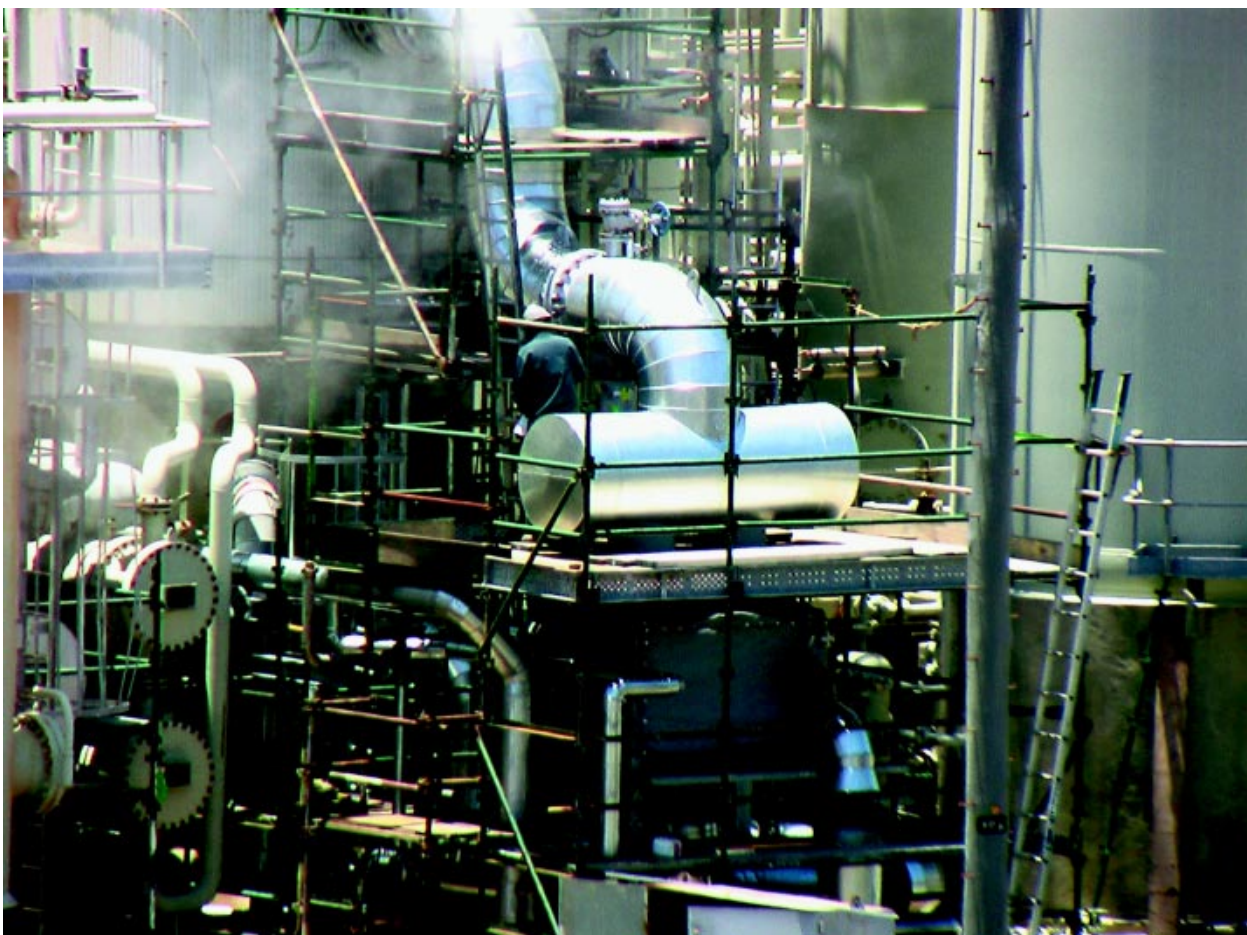
Fig. 4 One CPHE operating since 2006 as naphtha reboiler in an Australian refinery.
