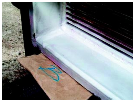
Fig. 10 Photo showing the result of the dye-penetrant test after a corner weld has been TIG repaired.
