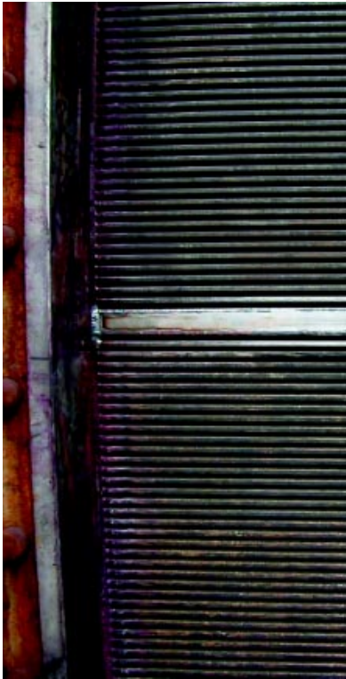
Fig. 12 Photo showing a cross-leaking CPHE channel sealed with a metal-strip
