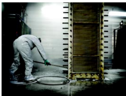
Fig. 7 Photo showing the un-restricted channels formed by the 45-degree angle plate pattern and the flat channels along the edges for draining. This means the hydro-jet passes through the heat-exchanger when the nozzle is tilted in 45 degree angle.
