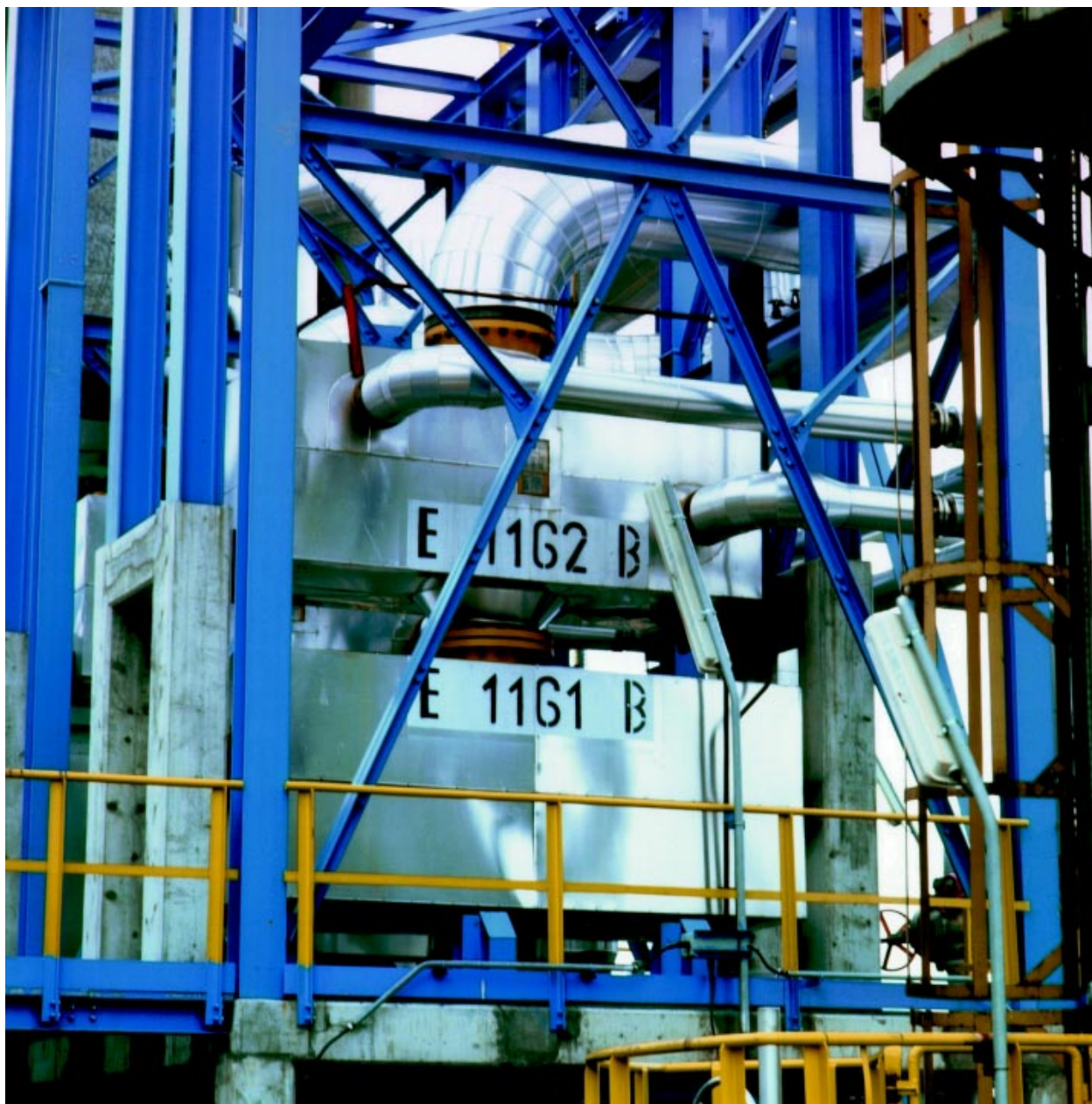
Fig. 5 Two out of four CPHEs operating since 1997 as ADU overhead vapour condensers in a European refinery.
